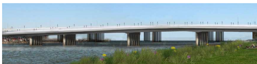
Artist's rendering of a future view of the bridges looking northwest from the eastern side of the Anacostia River.
